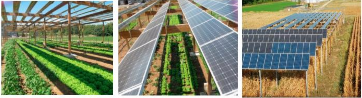
(a) Structure 4 m above the ground (b) Mono-crystalline PV arrays (c) Single-axis sun tracking system
