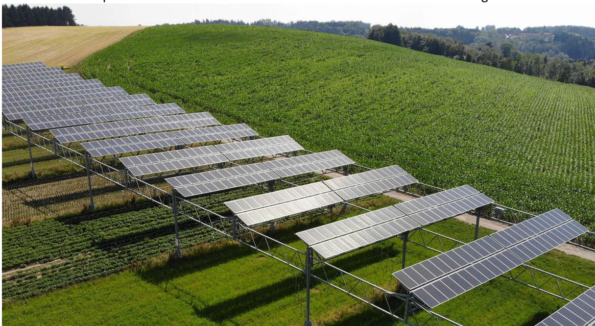
Image: The Agrivoltaic plant near Lake Constance in Heggelbach, Germany. Double usage of agricultural areas allows photovoltaics to be installed over fertile areas without eliminating these resources.
